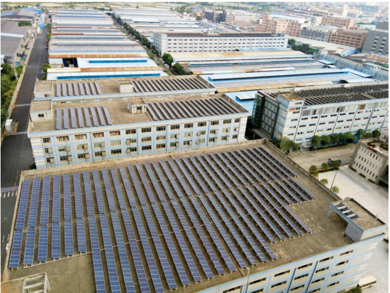
Solar PV Panels on the Roofs of Lesso Plants 聯塑廠區屋頂太陽能光伏板
